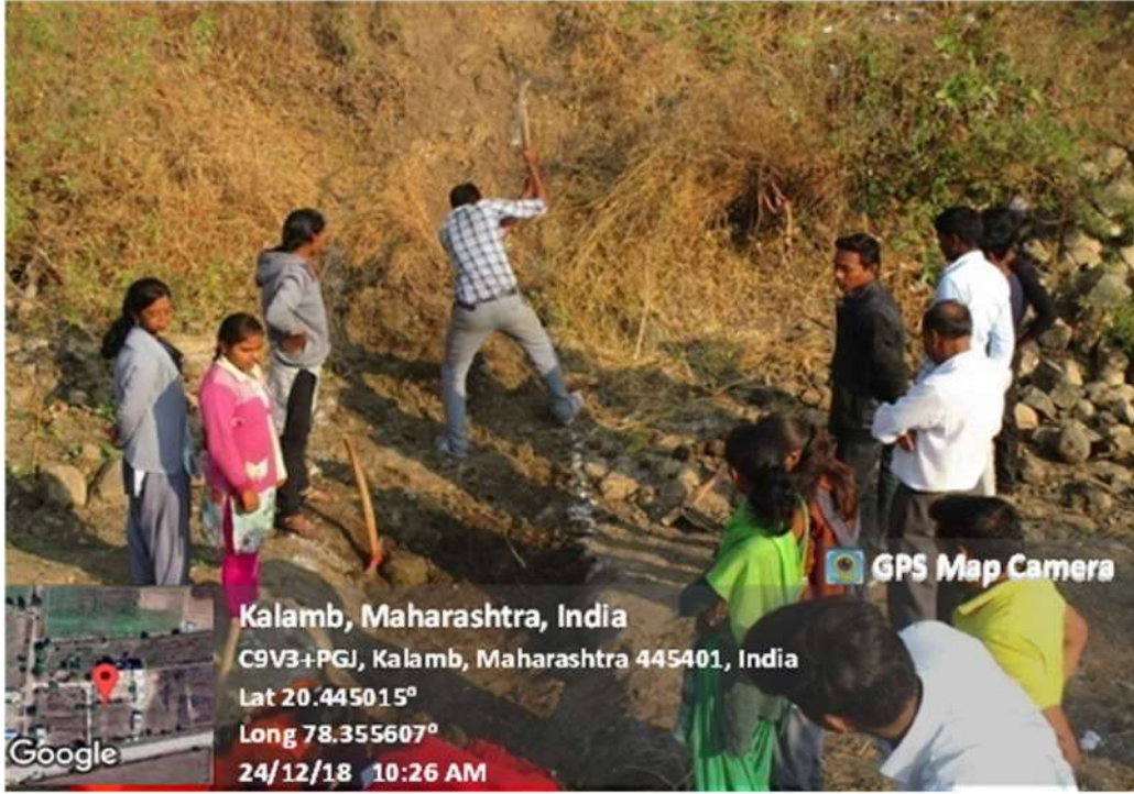
Snapshots During the Construction of Bund
